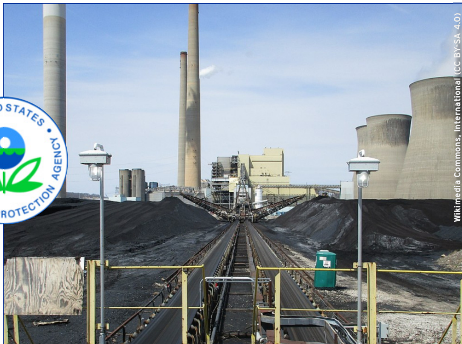
The John Amos Power Plant in West Virginia. Coal is being transported by conveyor belt into the facility where it will be pulverized.
